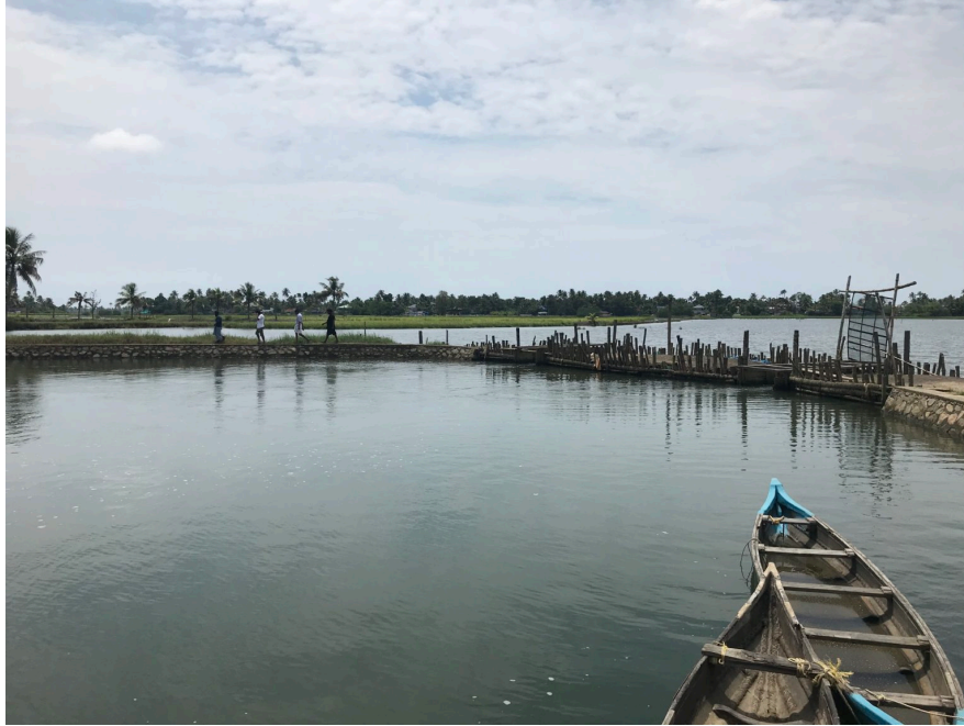
Figure 3. Sluice gate. Image by author.
