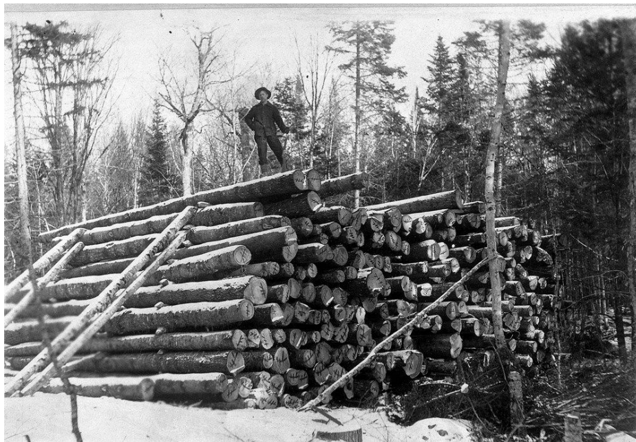
Image 8. "A large pile of logs made possible through parbuckling." (Source: published with permission from the Patten Lumbermen's Museum.)
