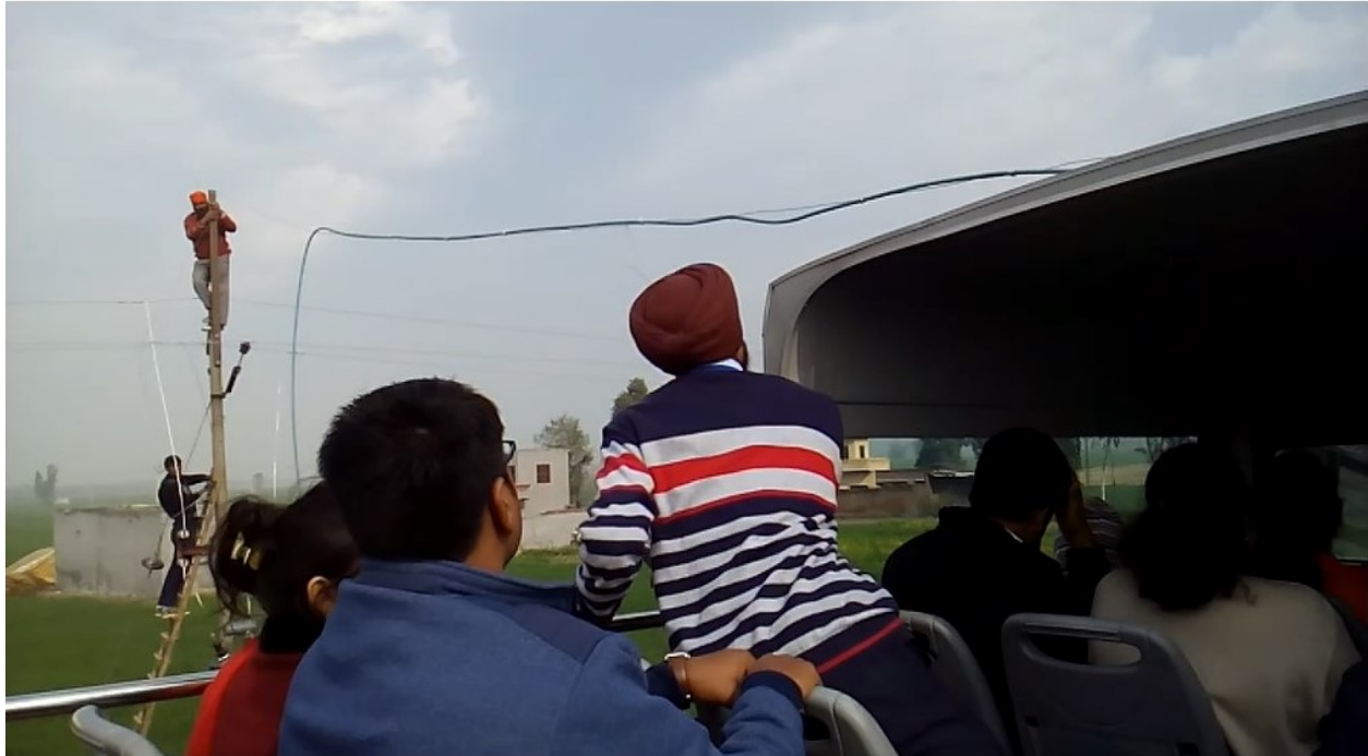
Figure 3. Men lifting a low-hanging cable passing over a road so that a bus can drive underneath, in Amritsar, India (2017). (Source: Still from a video by Abigail Kay).
